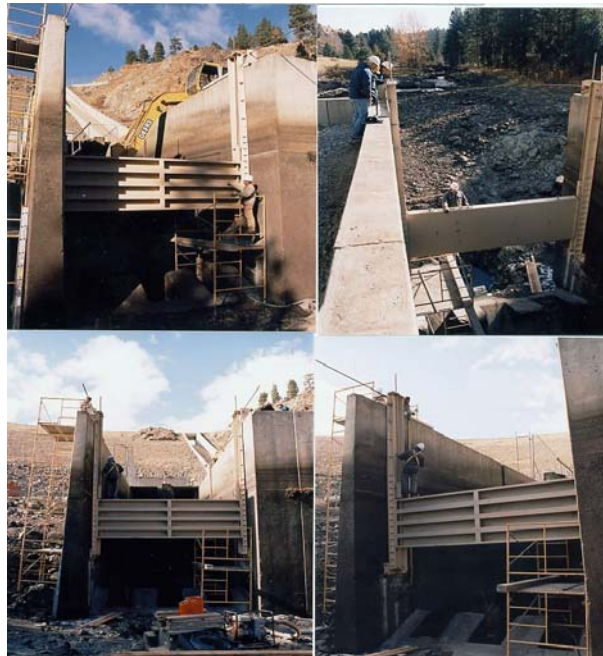
Figure 33. — Installation of first prototype deflector at Mason Dam in Oct 2002
