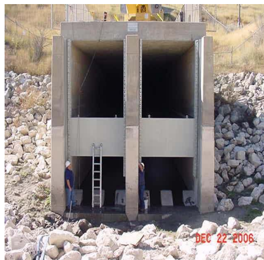
Figure 34. — Installation of Choke Canyon stilling basin deflectors in December 2006.
